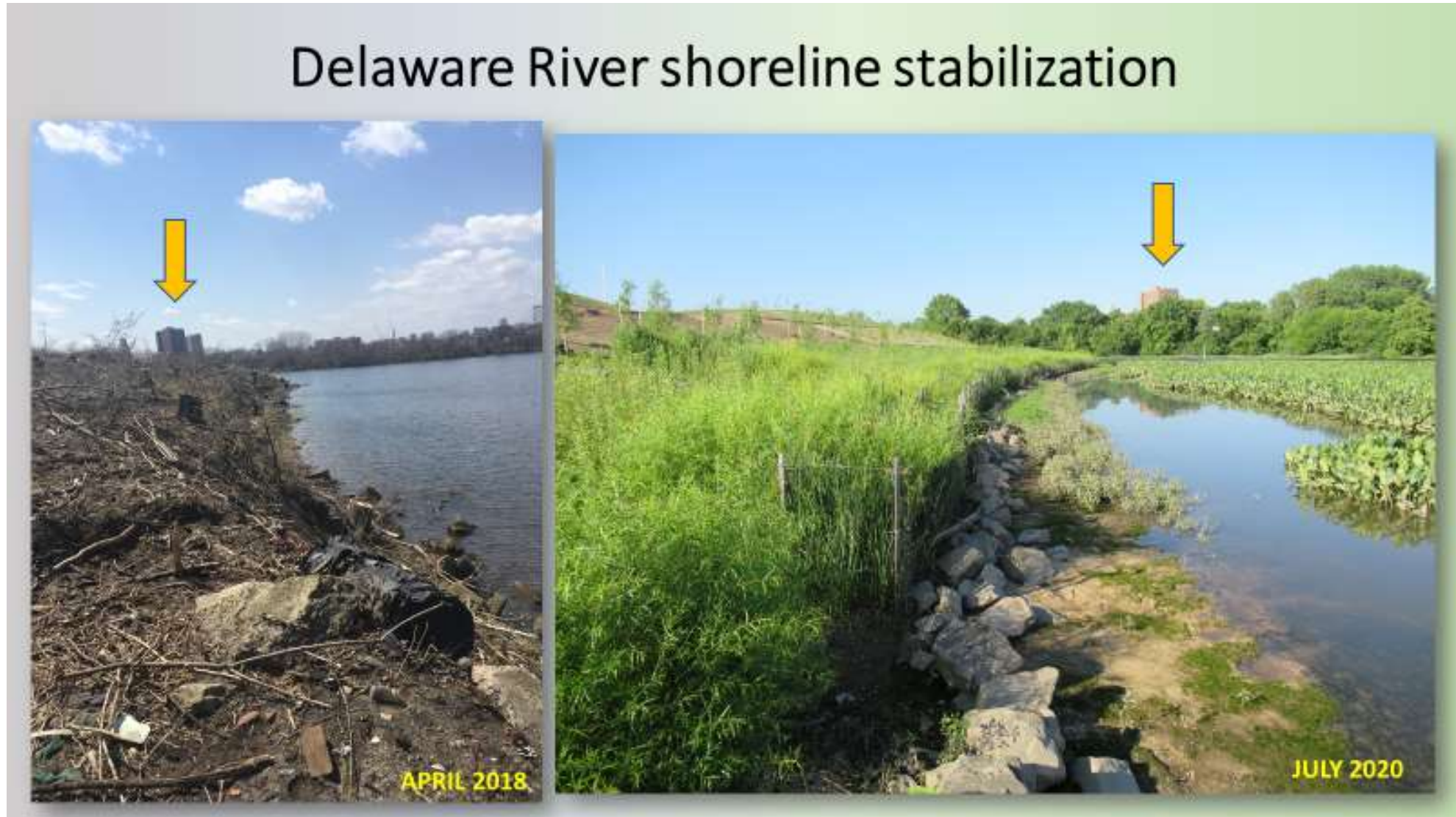
View south along Harrison Ave Landfill shoreline, showing solid waste at water's edge (right, 2018) and the stabilized shoreline (left, 2020), after solid waste relocation, with riprap and plantings (courtesy of NJDEP Office of Natural Resource Restoration).
