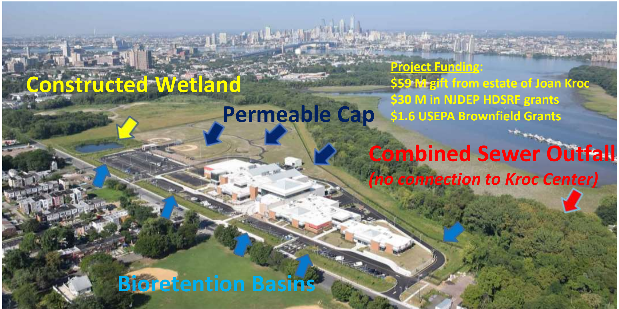
Aerial view toward southwest of Harrison Ave Landfill after remediation and construction into the Kroc Center, showing stormwater management features (2014).
