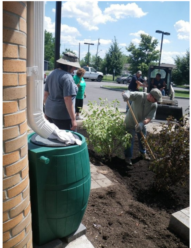
Building a demonstration rain garden.
